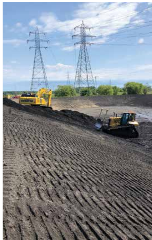
Ash being excavated from B.C. Cobb ash ponds in preparation for pond closure.
